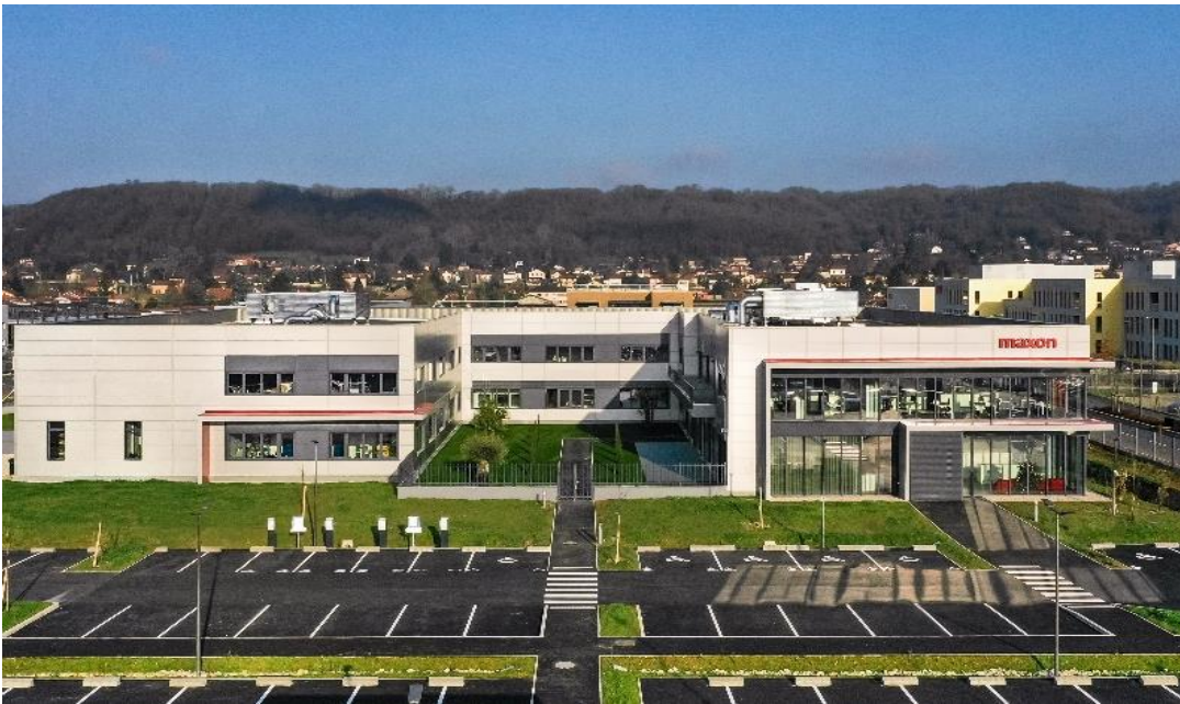
The Innovation Center at the new site in Beynost near Lyon. Image credit: maxon
