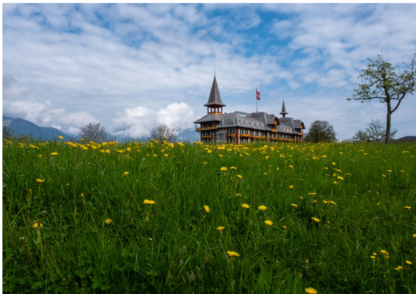
The Art Nouveau Hotel Pax Montana in Flüeli has been around for over 130 years and is now a protected historical monument.
